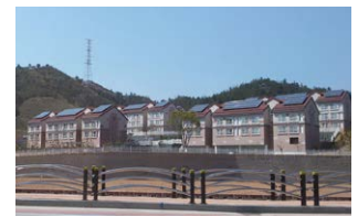
Daelim Industry (Korea's first boiler-less apartment)
