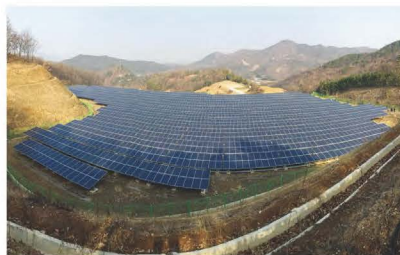
SechoJungri PV Power Plant
