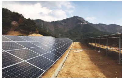
Koheung Solar Farm
