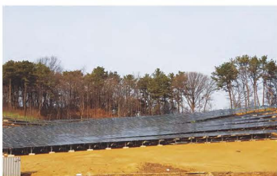
Ilpori PV Power Plant
