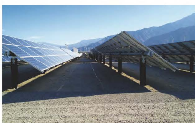
Keokun PV Power Plant
