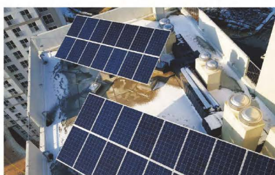
Incheon Building Roof
